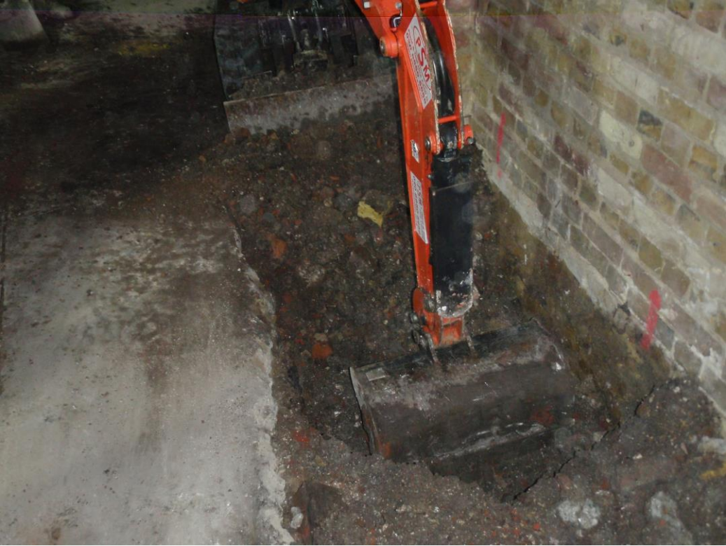
Plate 2. View of foundation pad trench (looking NW)
