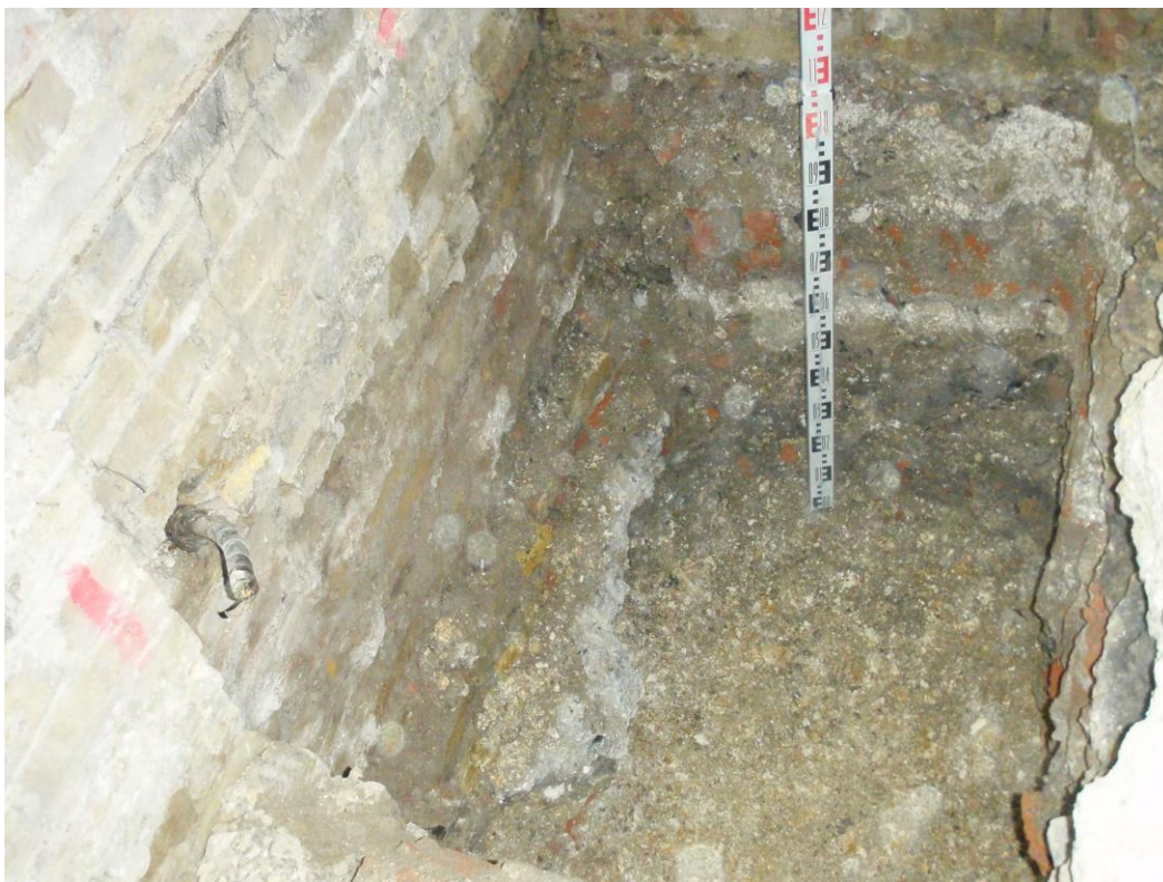
Plate 4. Foundation pad trench (looking NE)
