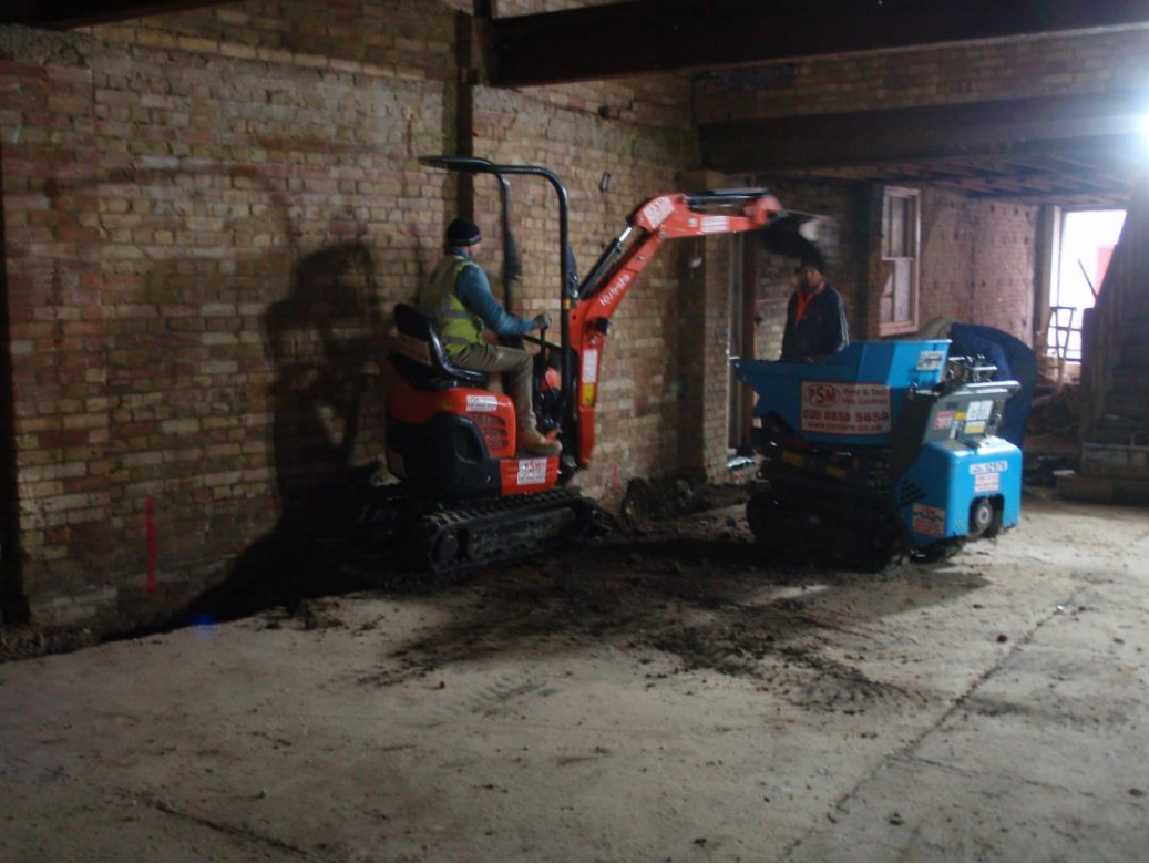
Plate 1. View of the site (looking NE)
