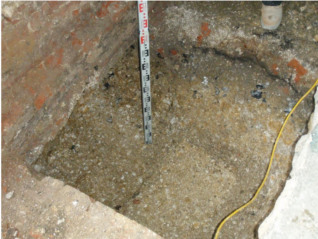
Plate 3. Foundation pad trench (looking NE)
