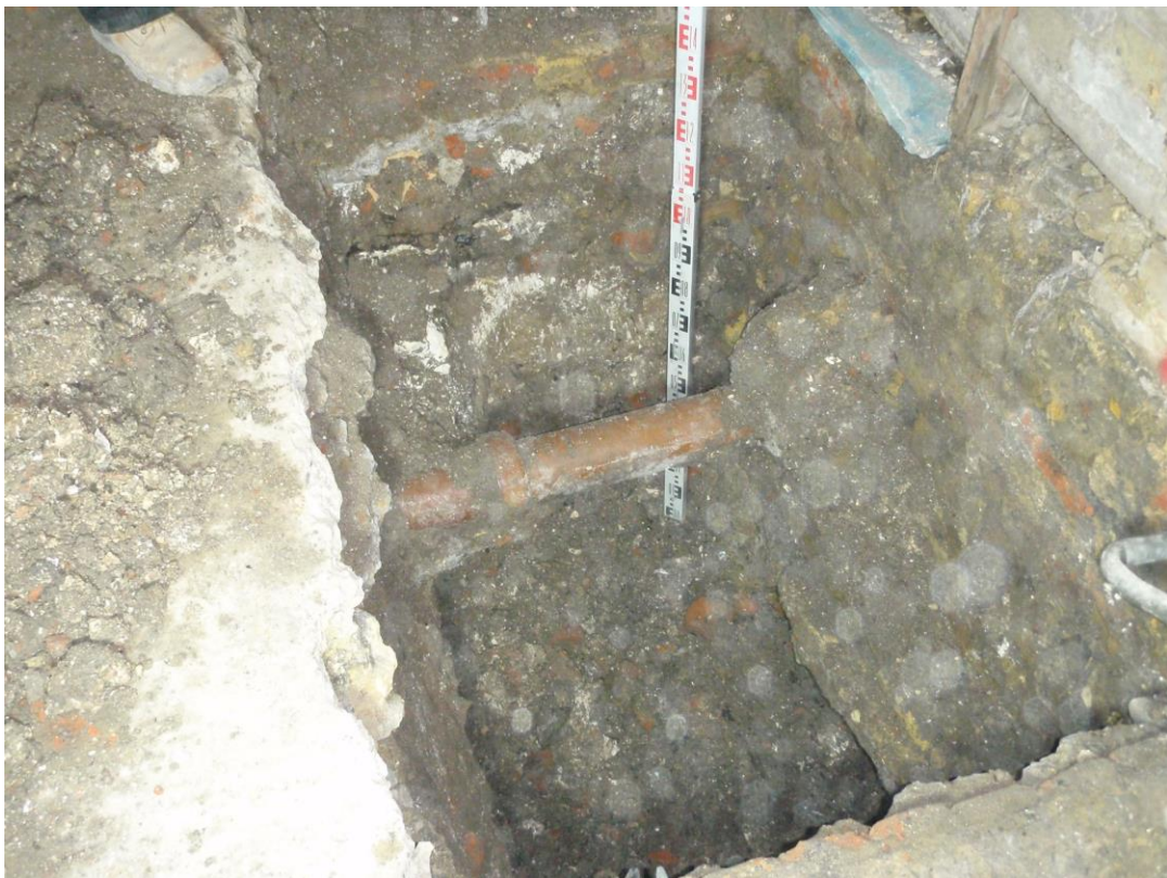
Plate 6. Foundation pad trench (looking NE)
